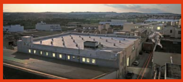
The new soft drinks factory now in its final stages.
